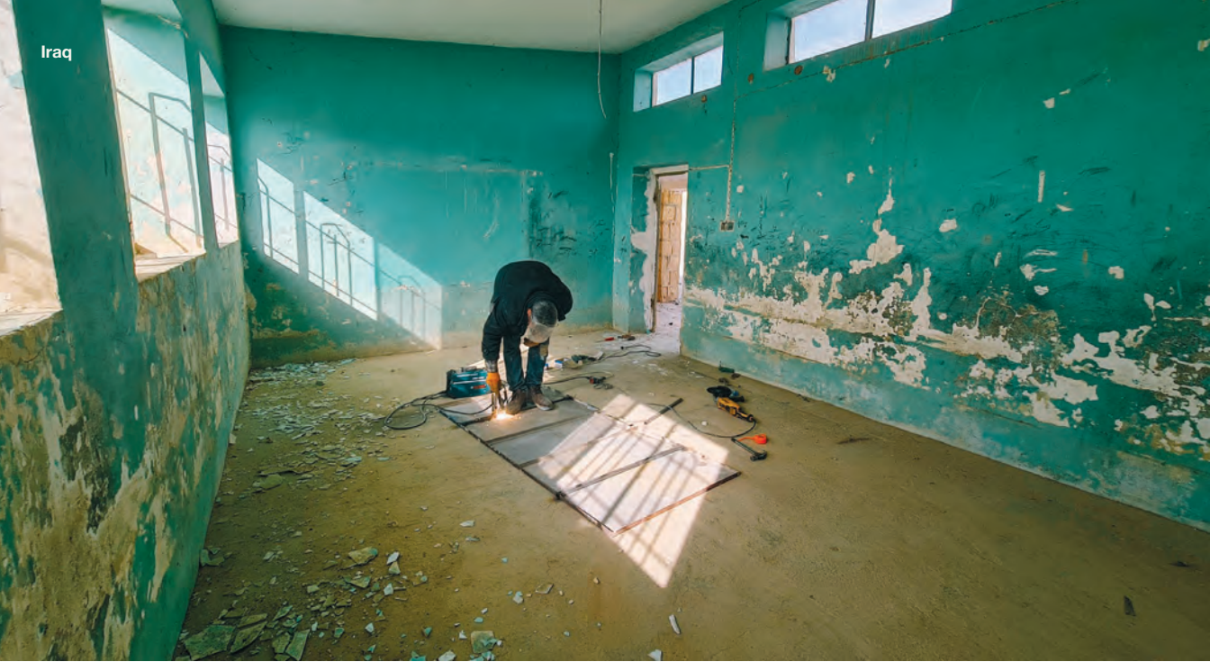
Iraq School Rebuild - In Progress March 2021
